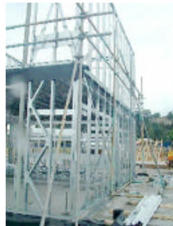
This is the underside of a floor. The joists are constructed in a lattice format which therefore means obviously, as I said earlier, that all services can be passed through easily. There are service holes in the cross members and those holes there are purely for lifting purposes, in other words the crane can actually be used to lift the cassettes in place and those holes are sealed when the house is finished.
